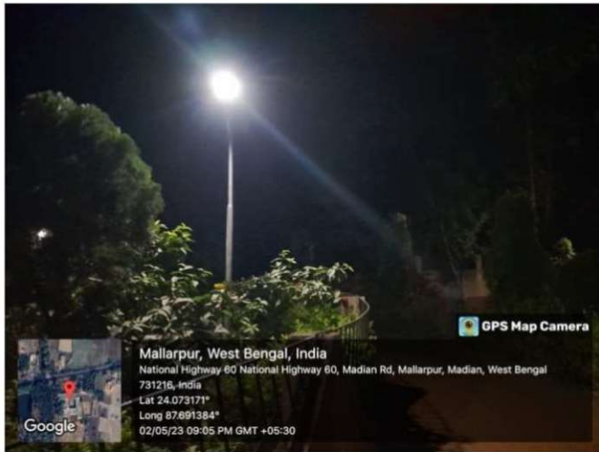
Figure 1a: The street light has been installed inside the Butterfly Garden situated in front of the institution.
