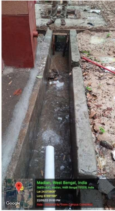
Fig 5: Rain water flowing into recharge chamber.
