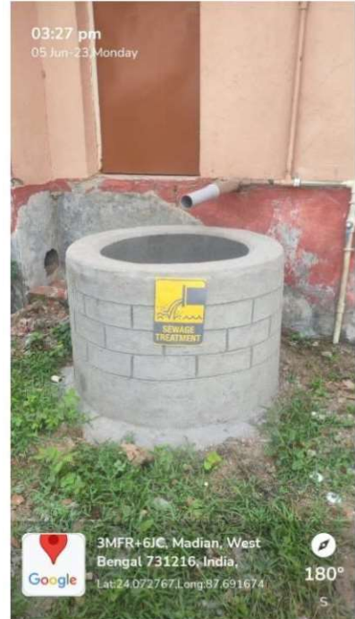
Fig 7.3: Liquid waste pit
